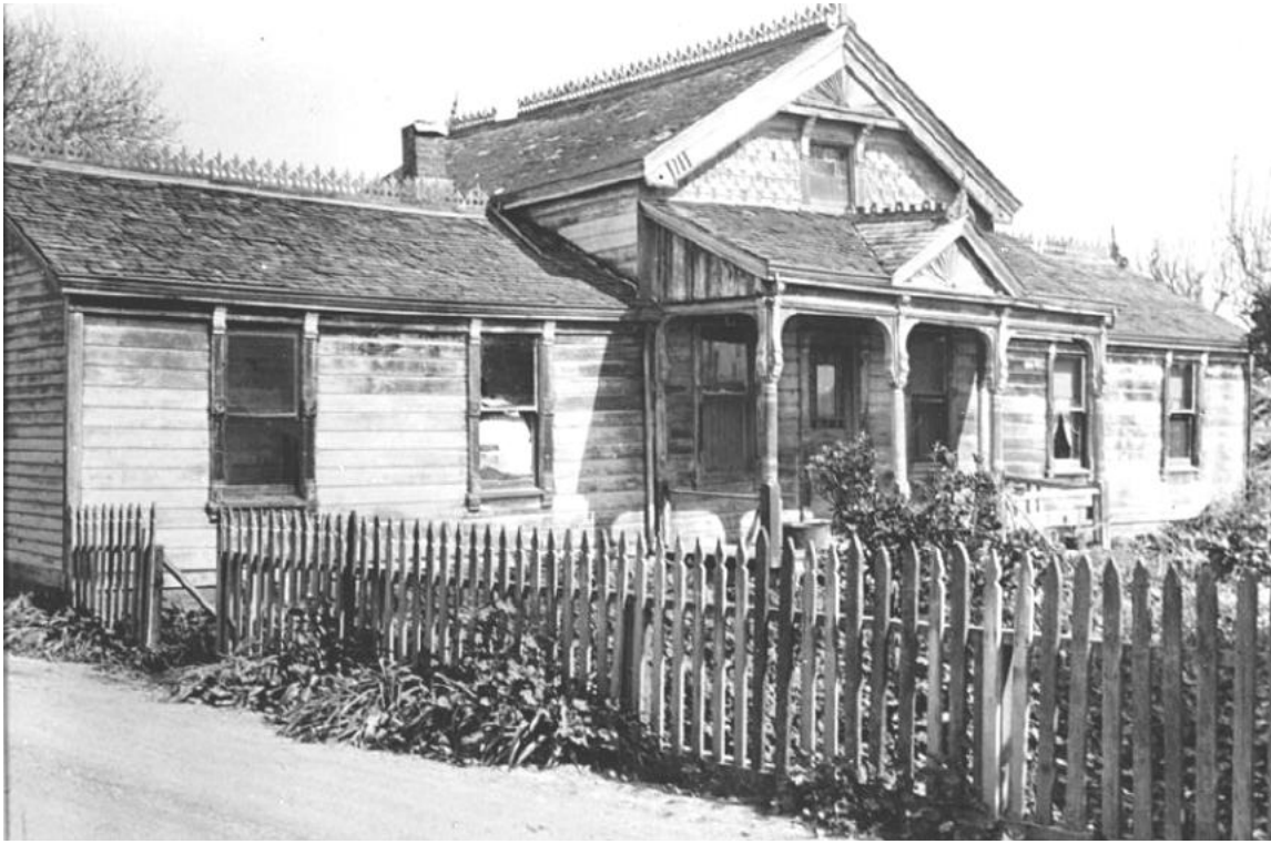
The old Henry Smith home at the end of Vallejo Street. Built in 1852 by Henry Clay Smith it is shown here in a derelict state shortly before the end of its life, but the glory and craftsmanship of the old building can be clearly seen.
