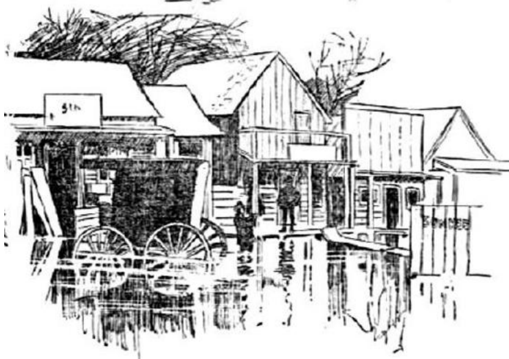
Alvarado's Chinatown during the flood.
