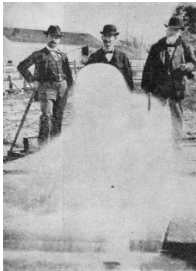
(Left): Artesian well at Alvarado belonging to the Oakland Water Co. bored in 1894.
