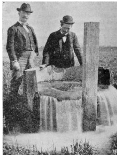
(Left): Artesian well at Alvarado belonging to the Oakland Water Co. bored in 1894.
