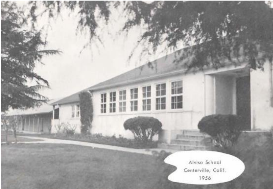
The new Alviso Grammar School was finished in October 1940.
