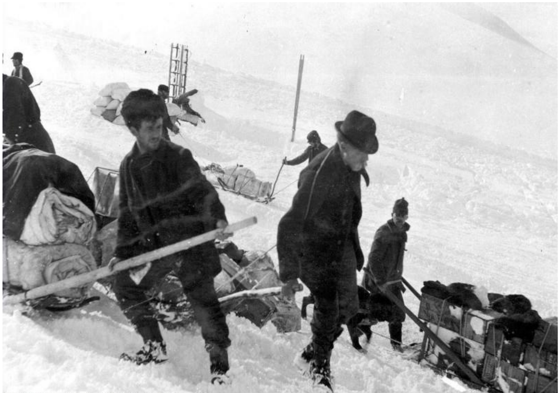
DESCENDING DOWN THE EAST SLOPE OF THE CHILKOOT PASS
