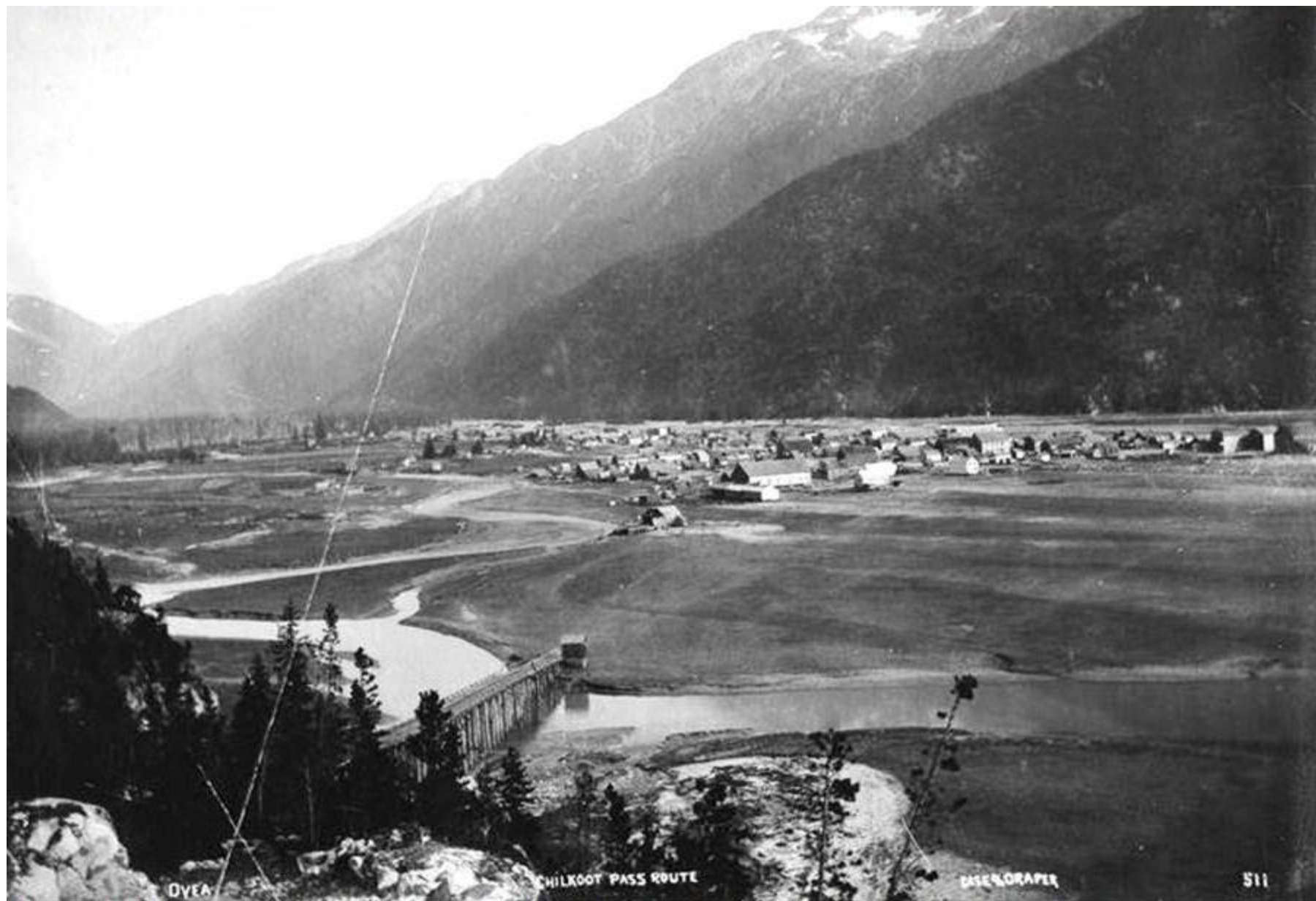
THE OLD DESERTED VILLAGE OF DYE A AT THE HEAD OF LYNN CANAL -- 5 MILES NORTH OF SKAGUAY, 1902.
