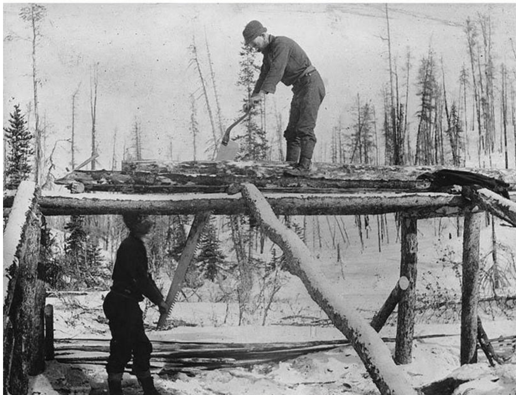
Two men whipsawing lumber, possibly at Bennett, British Columbia, ca. 1898.
