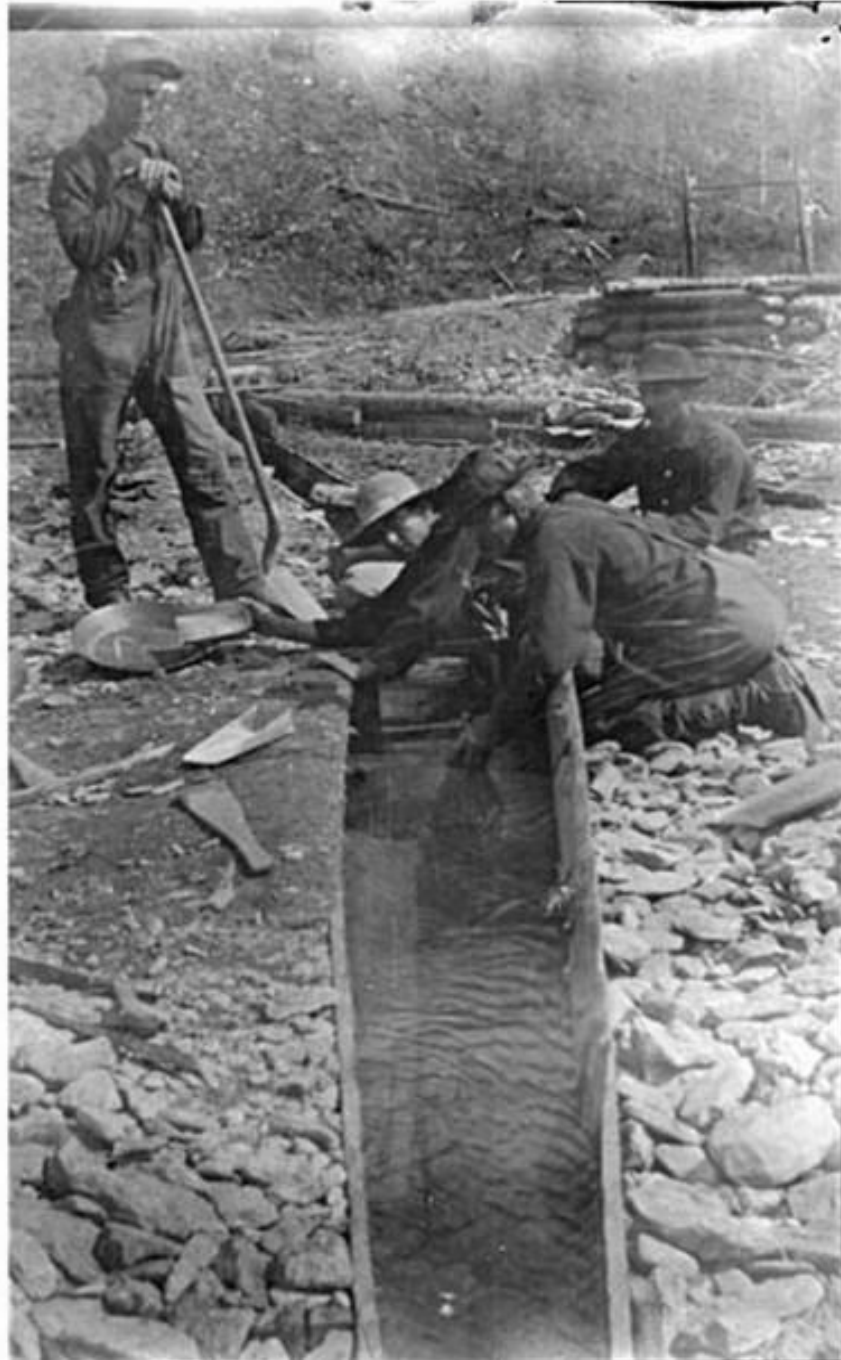
Mining operation showing four men with gold pan and sluice, Bonanza Creek, 1898
