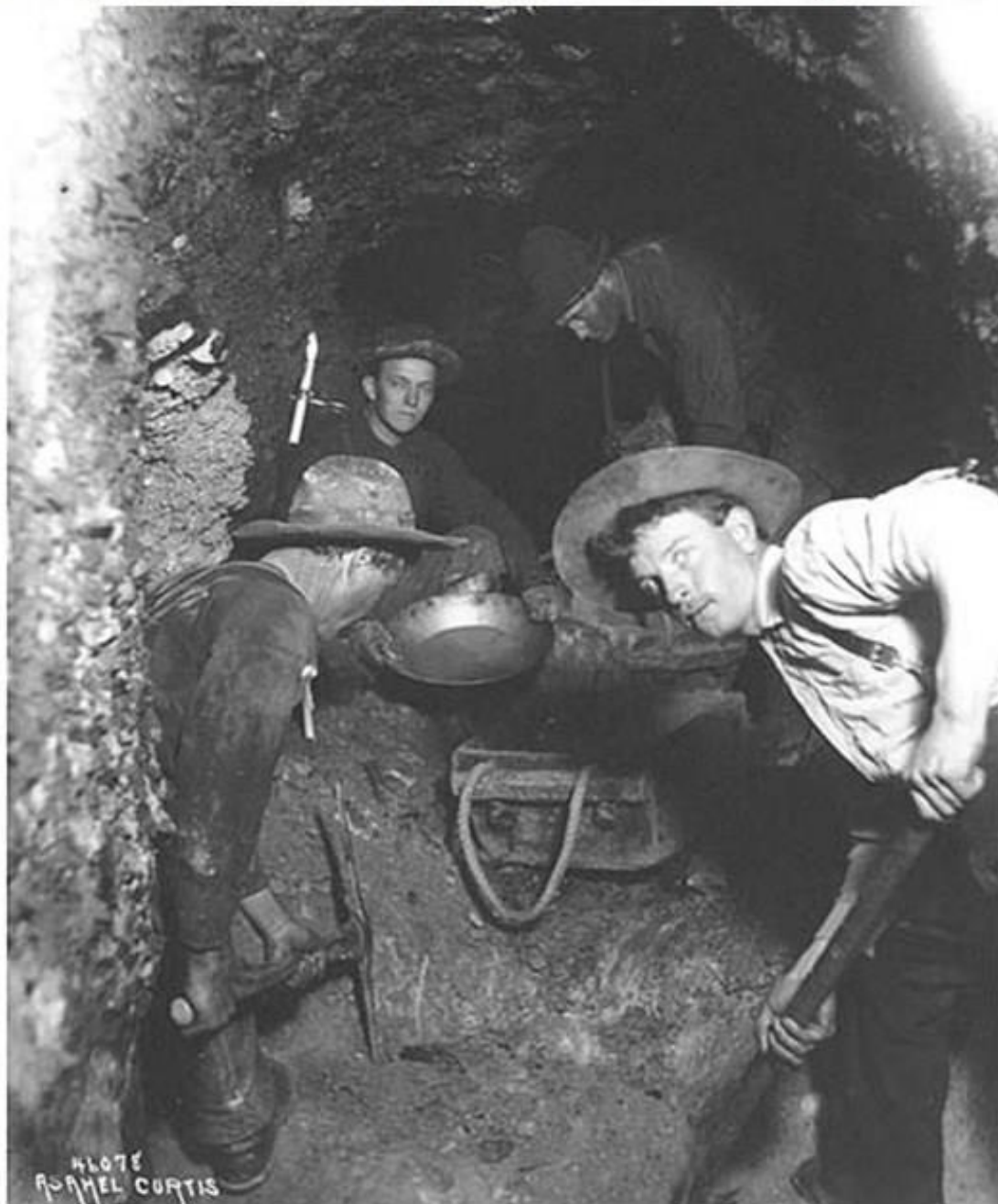
"Mucking thawed ground in a drift on 16 Eldorado," underground mining shaft in Yukon Territory.
