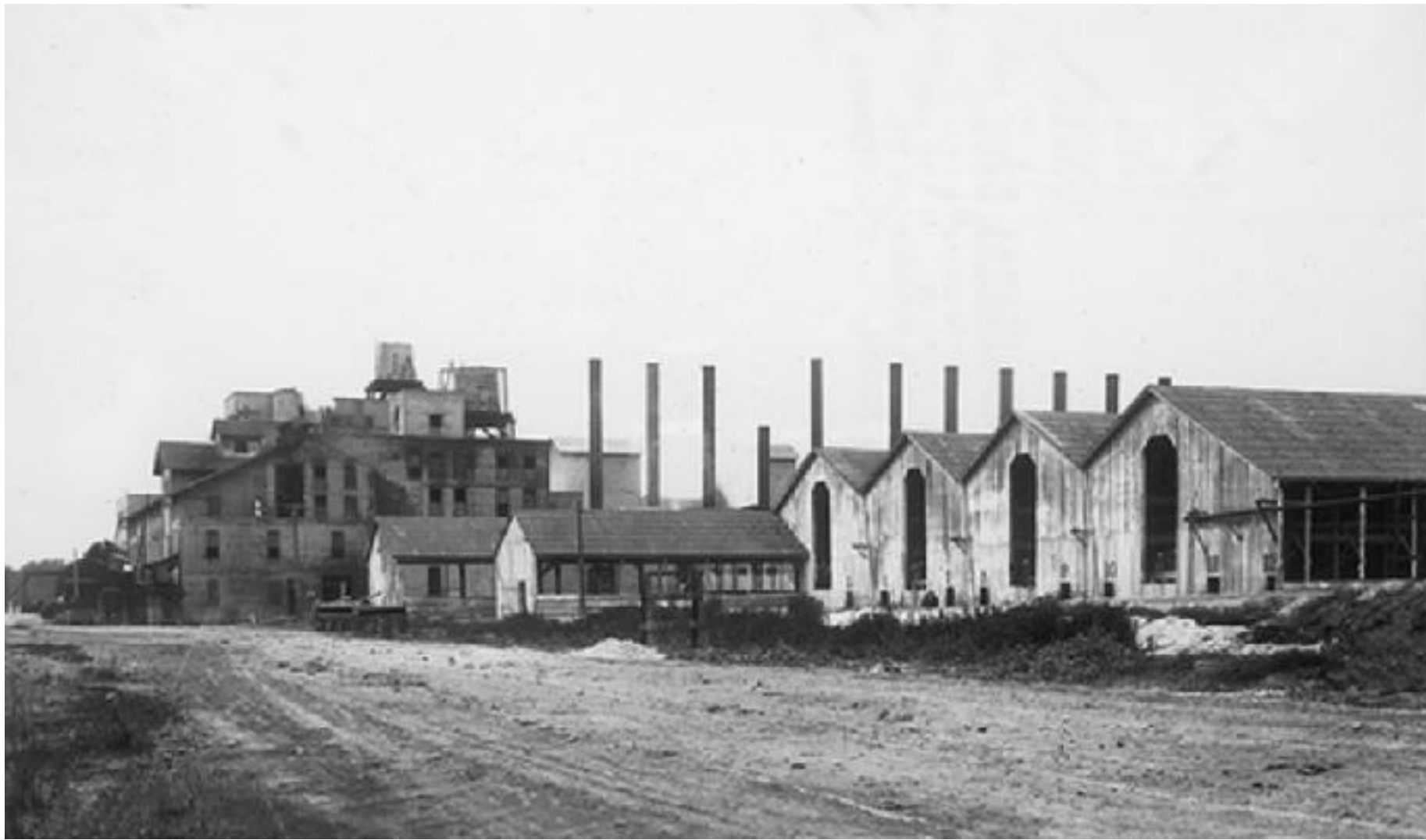
The Alameda Sugar Company as it looked at the time of the sale of the property in December 1926 to the Holly Sugar Company. The buildings were showing signs of great wear to the exterior and within ten years had to be replaced with new construction. Note the number of smoke stacks, each boiler had its own smoke stack. When the old buildings were replaced with new construction in 1936, one 204-foot smoke stack would replace the eleven that had previously existed.
