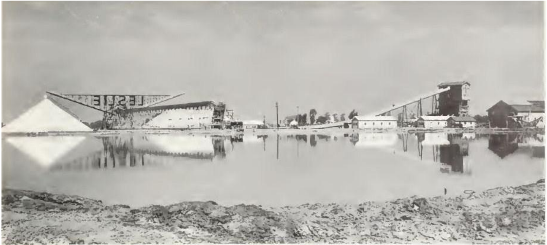
Leslie Salt crude plant at Baumberg (south of Mt. Eden). The pond area, which includes most of the important 19th century salt works, is 4,630 acres. The washer (center) has a design of 180,000 tons a year. Bulk shipments only are made from the bunker (right).
